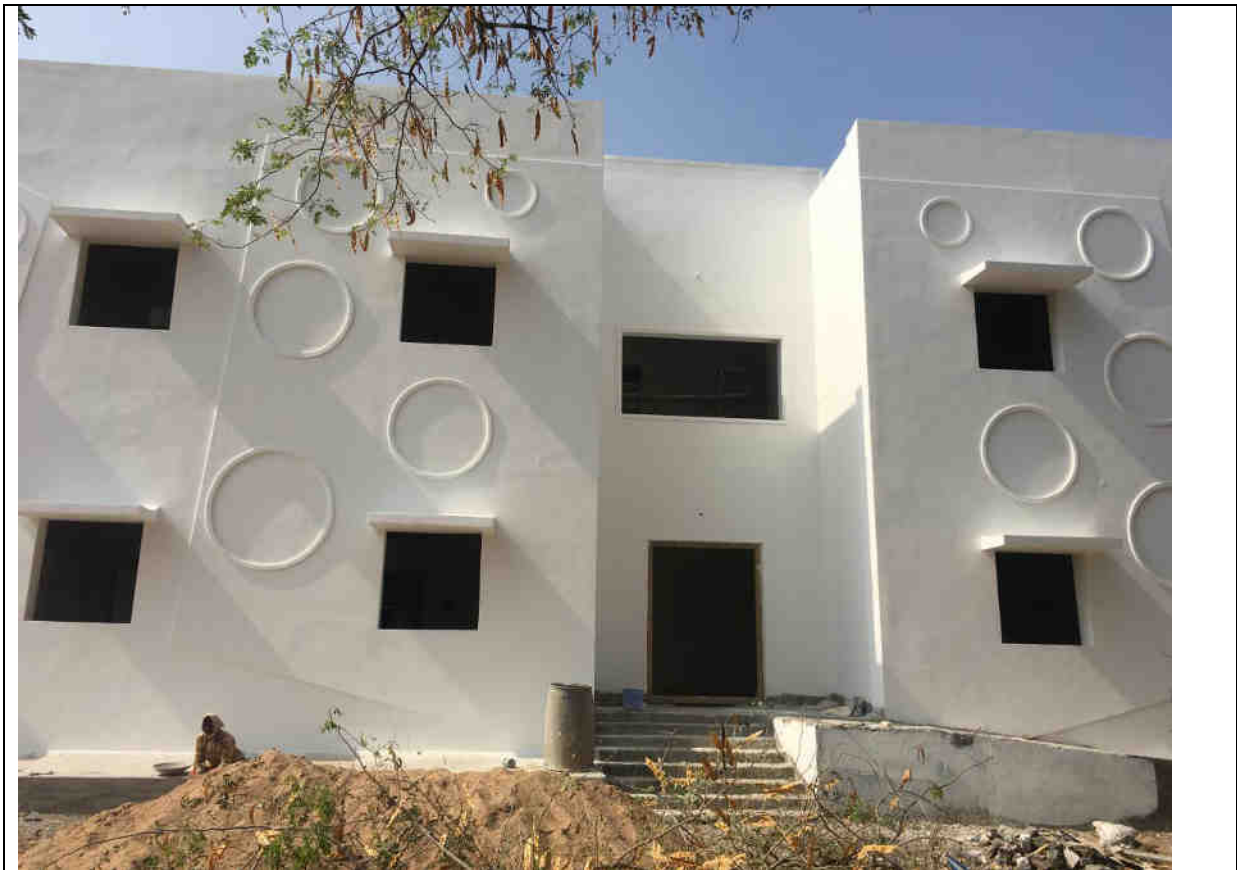
Hostel Block Front view
