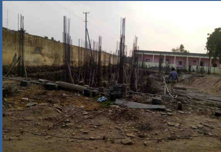
Science Block under construction
