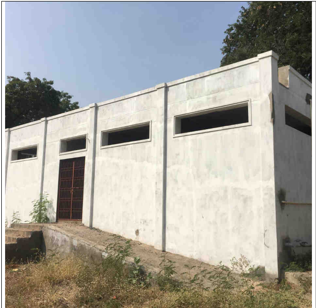
Women Toilets Block Side View
