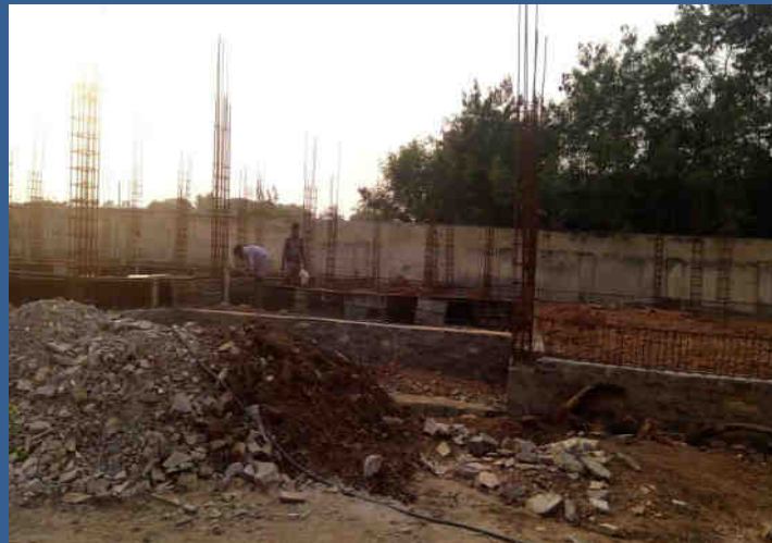
Library under construction
