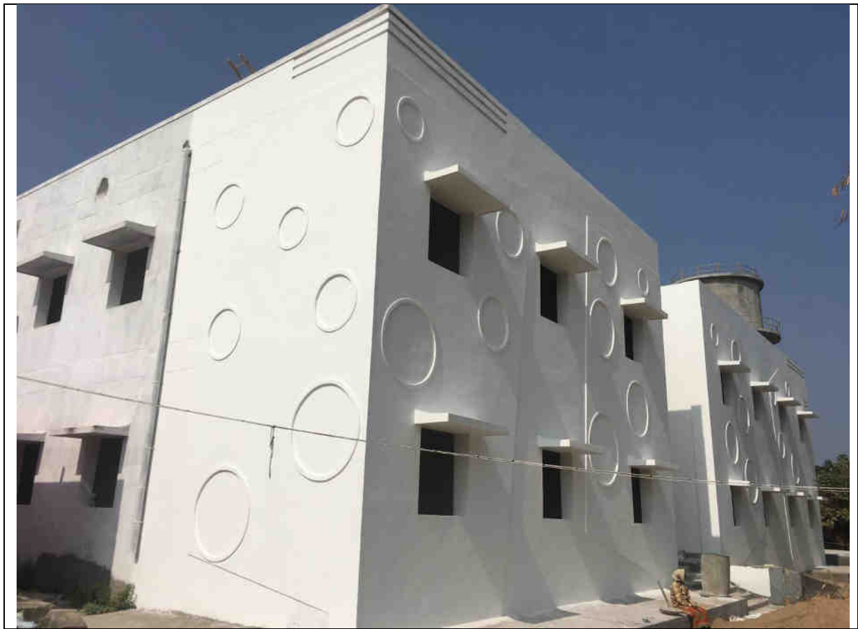
Hostel Block Side View
